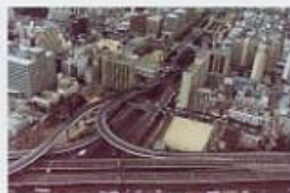
生田川出入口付近 Around the Ikutagawa On and Off Ramps
