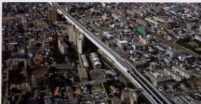
復旧後 Restored bridge
