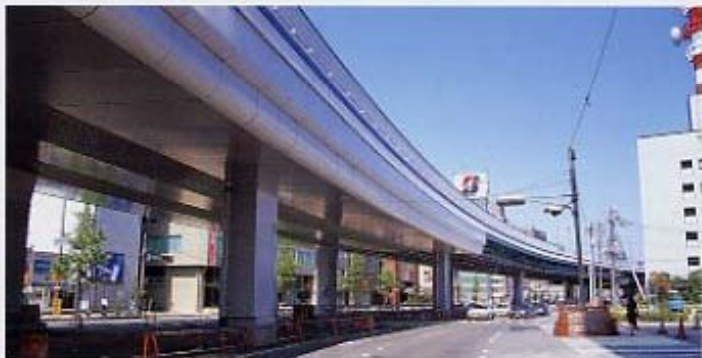
復旧後 Restored viaduct
