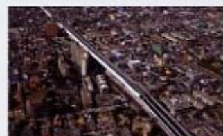
復旧した神戸市東灘区深江本町付近 Reconstructed town and the expressway in Fukae-honmachi, Higashinada-ku, Kobe
