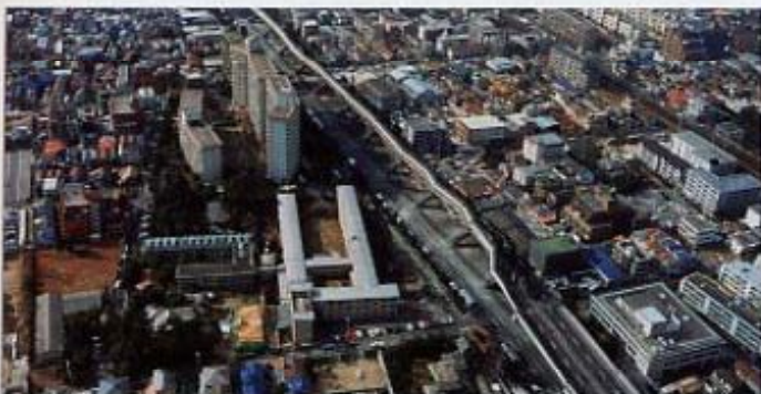
震災直後 Immediately after the earthquake
